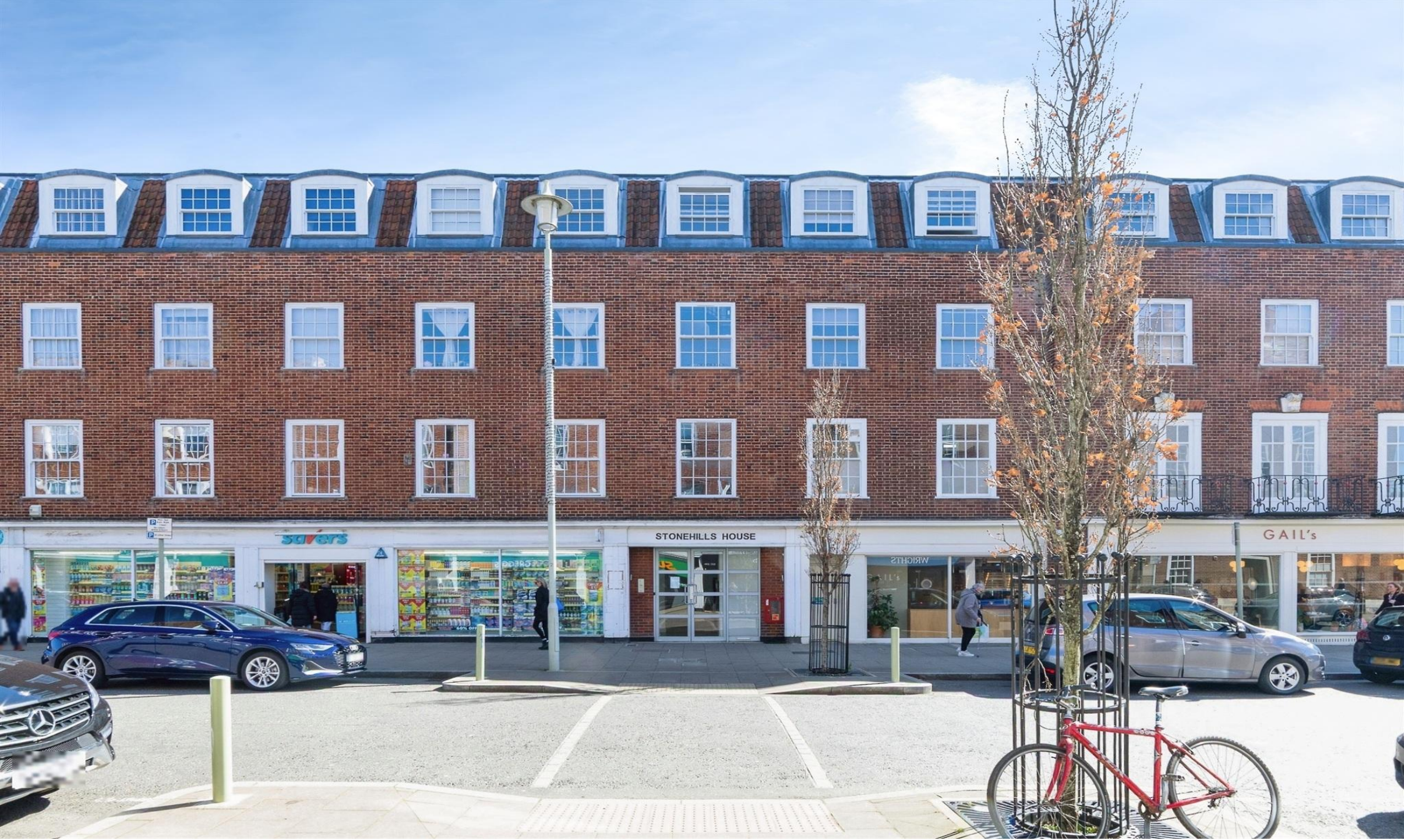
Stonehills House Stonehills, WELWYN GARDEN CITY AL8 6DL
