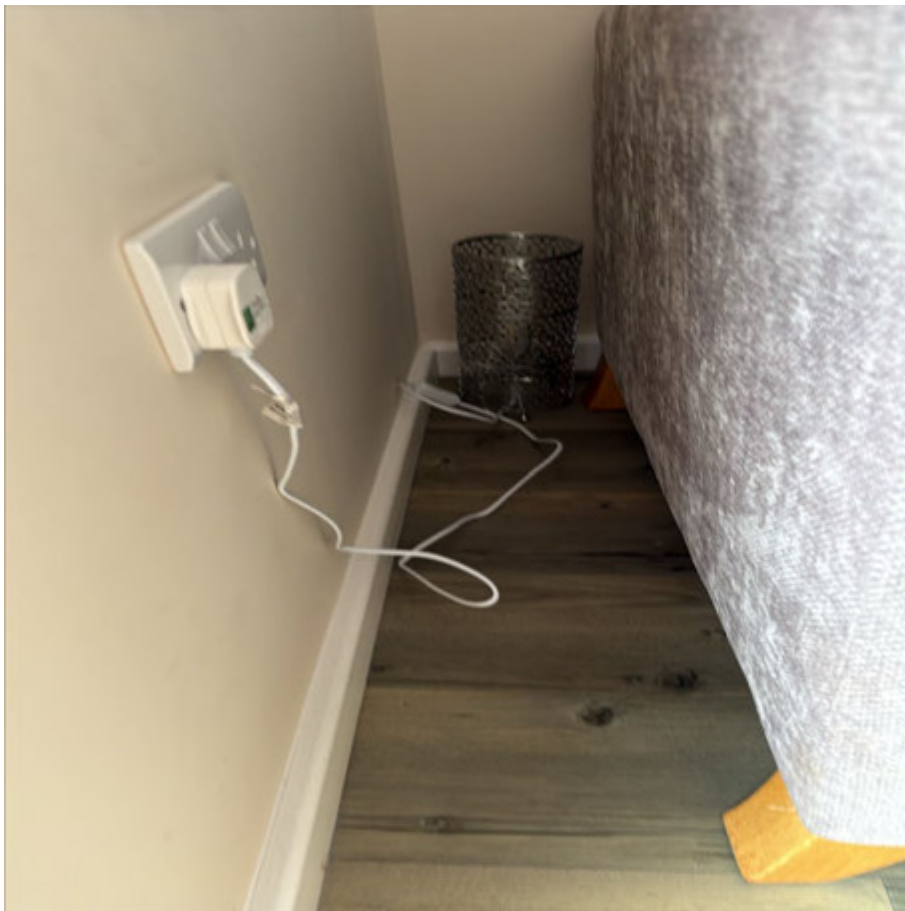
Living Room – 1 no. floor standing light
