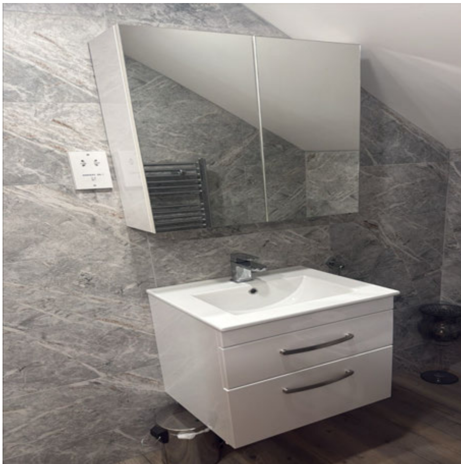
Bedroom 1 En Suite – The next three pictures show the mirrored cabinet, chrome tap and waste, two draw vanity unit, shower, toilet waste bin, and chrome towel rail
