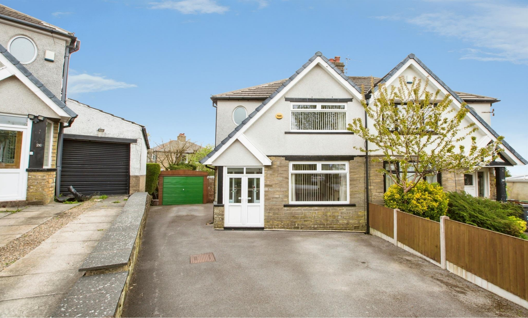
Mount Avenue, HALIFAX HX2 0LF
