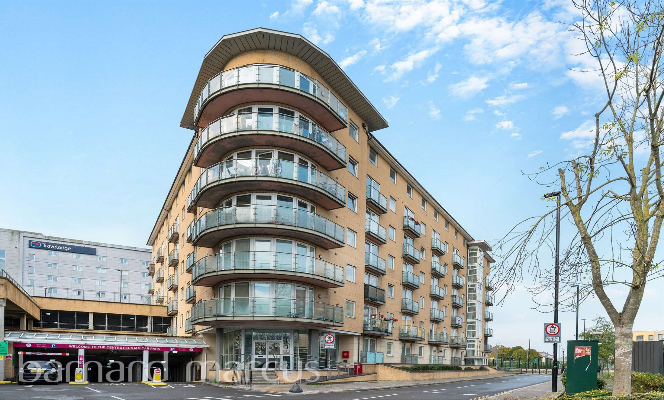
Bergenia House Bedfont Lane, Feltham TW13 4GE
