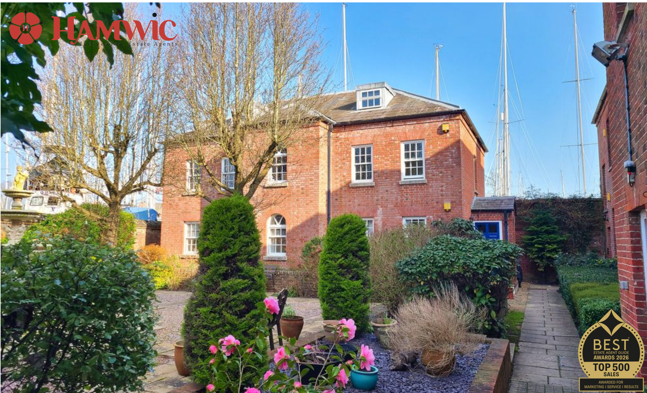
Frobisher Court, Maritime Avenue, SO40 Southampton
