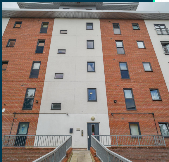
Light Building, Lumen Court, PR1
