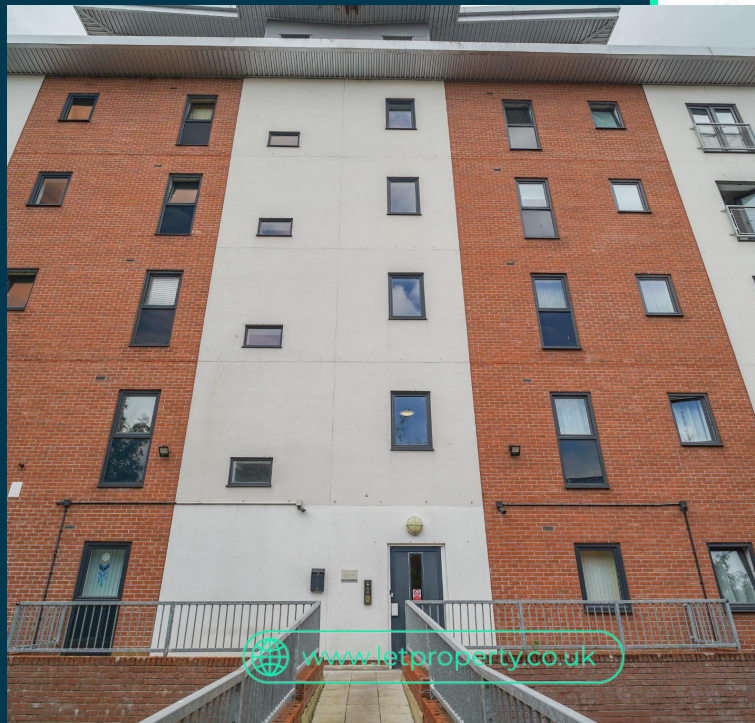
Light Building, Lumen Court, PR1
