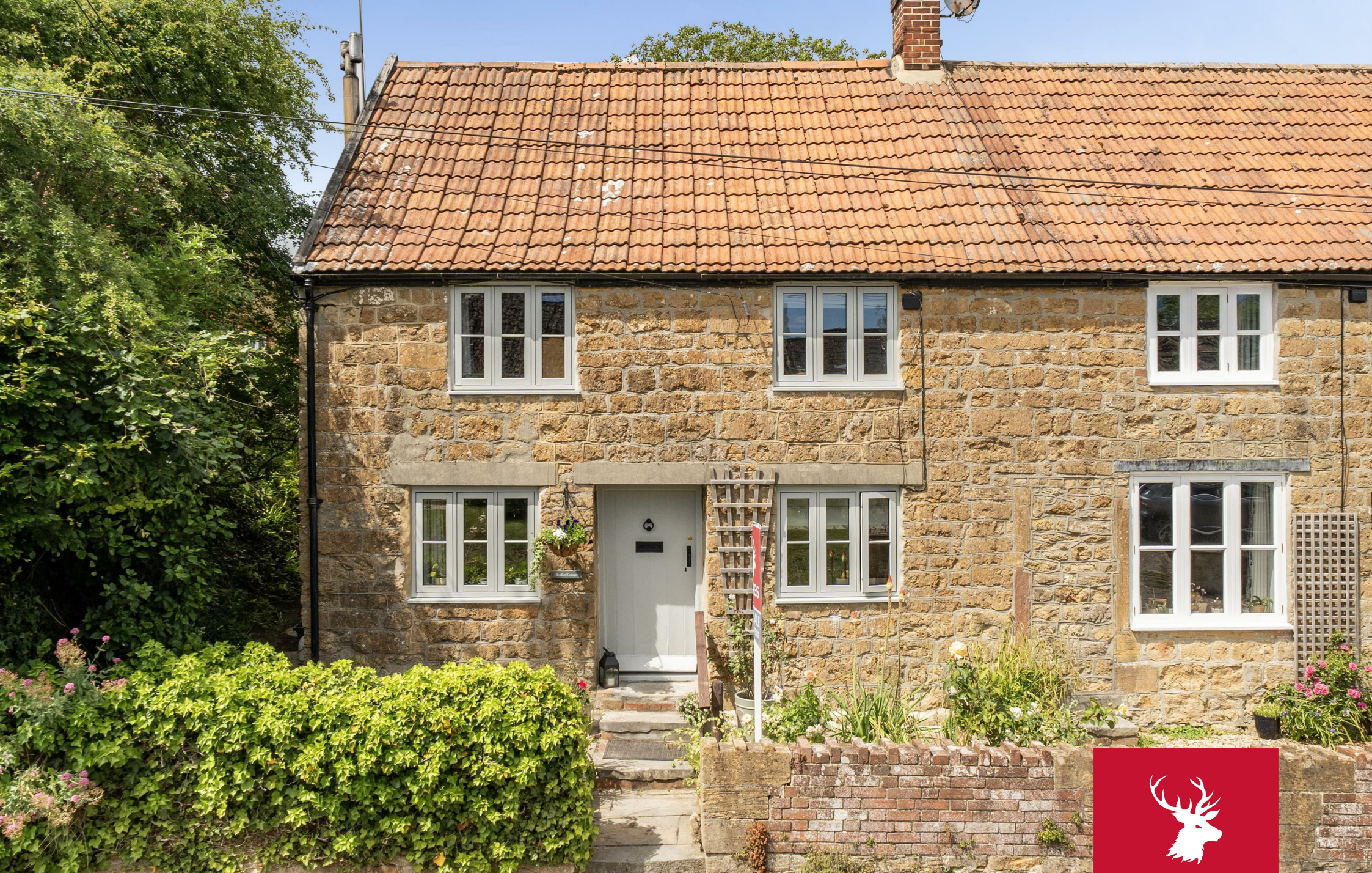
1 Bedford Cottages, Lambrook Road
