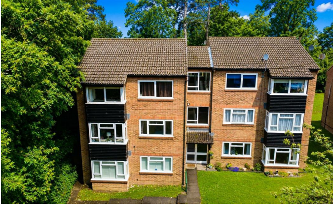
COMMUNAL ENTRY DOOR
