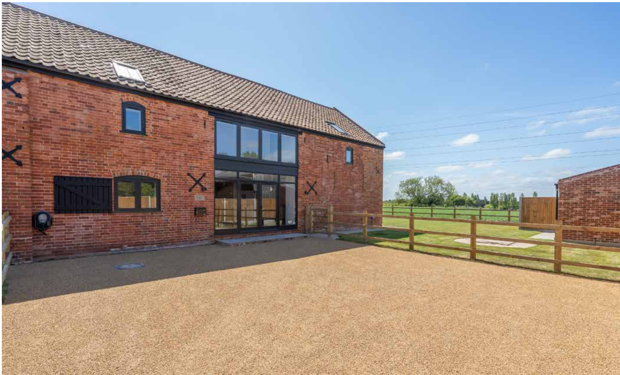
Pheasant Barn Rackhams Corner | Corton | Suffolk | NR32 5LB
