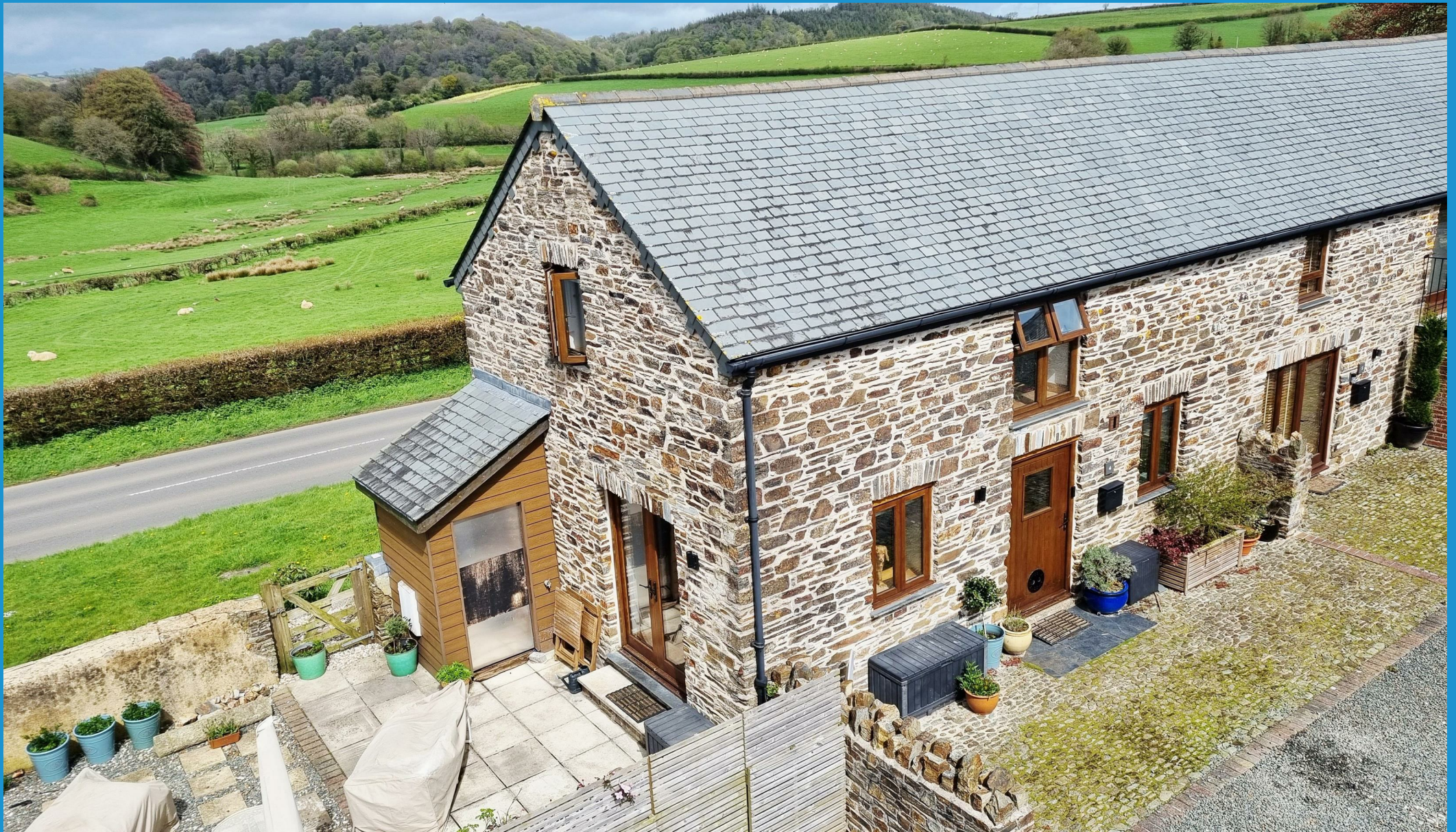
4 Warracott Court Chillaton Chillaton | Lifton Devon
