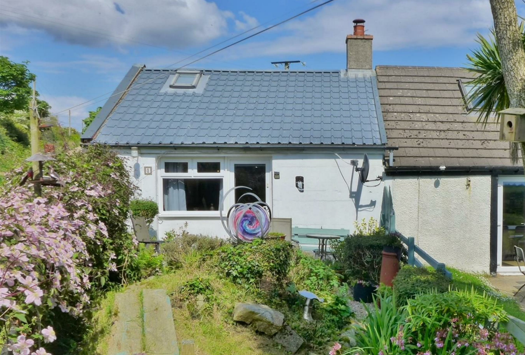
1 Bourtree Bank Cottage, Kilmory, Isle Of Arran, KA27 8PG
