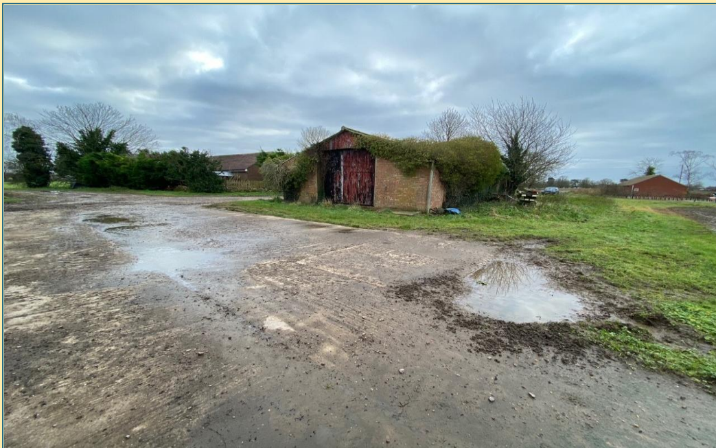
BUILDINGS TO BE DEMOLISHED
