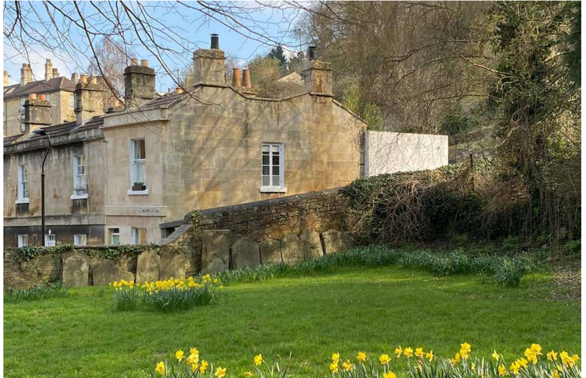
WEST ELEVATION IN CONTEXT FROM ALTON PLACE
