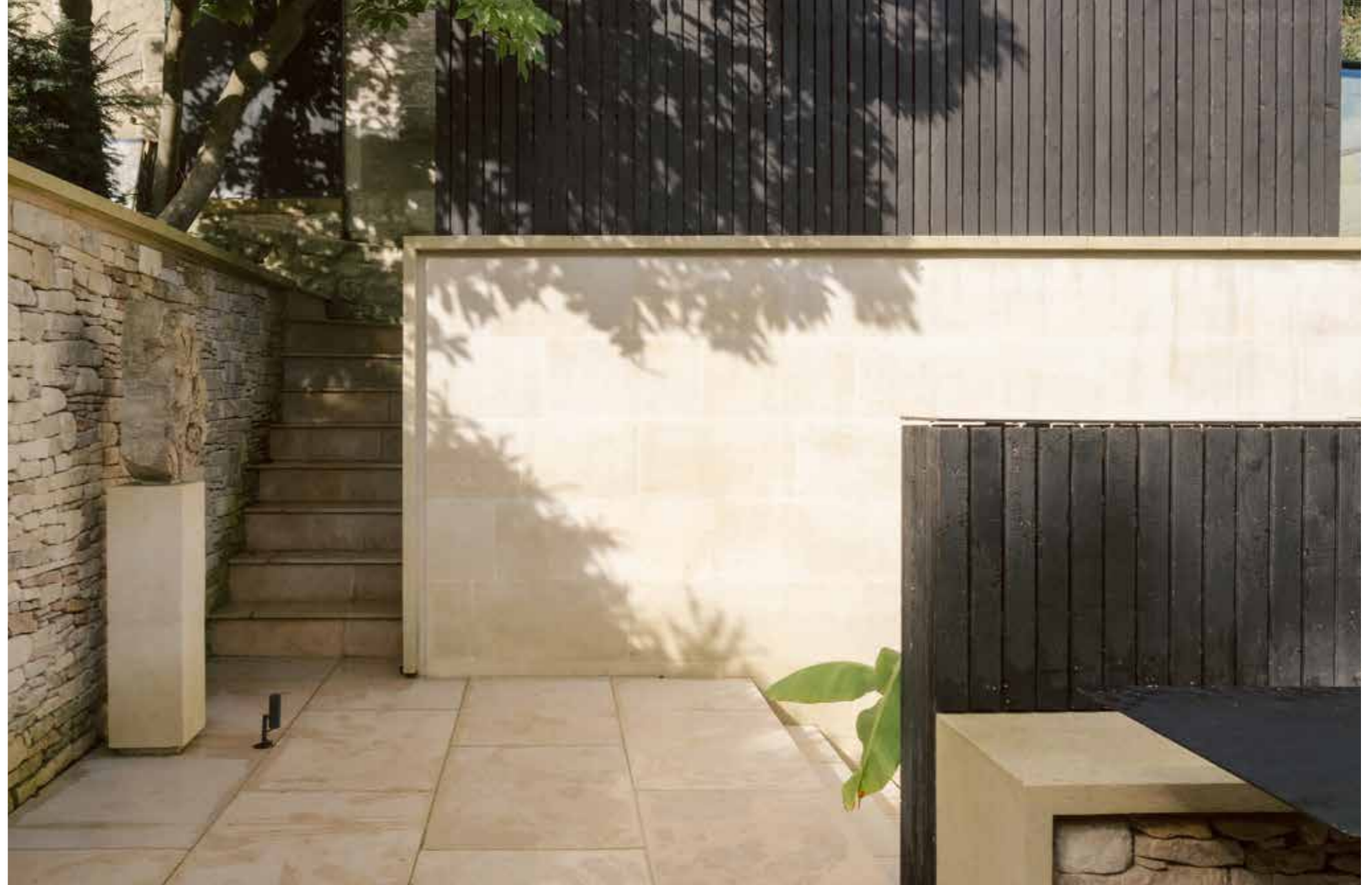
MIDDLE COURTYARD EXTERIOR VIEW WEST HIGHLIGHTING THE EXTERIOR LANDSCAPING & SEMI-SUBTERRANEAN EXTENSION
