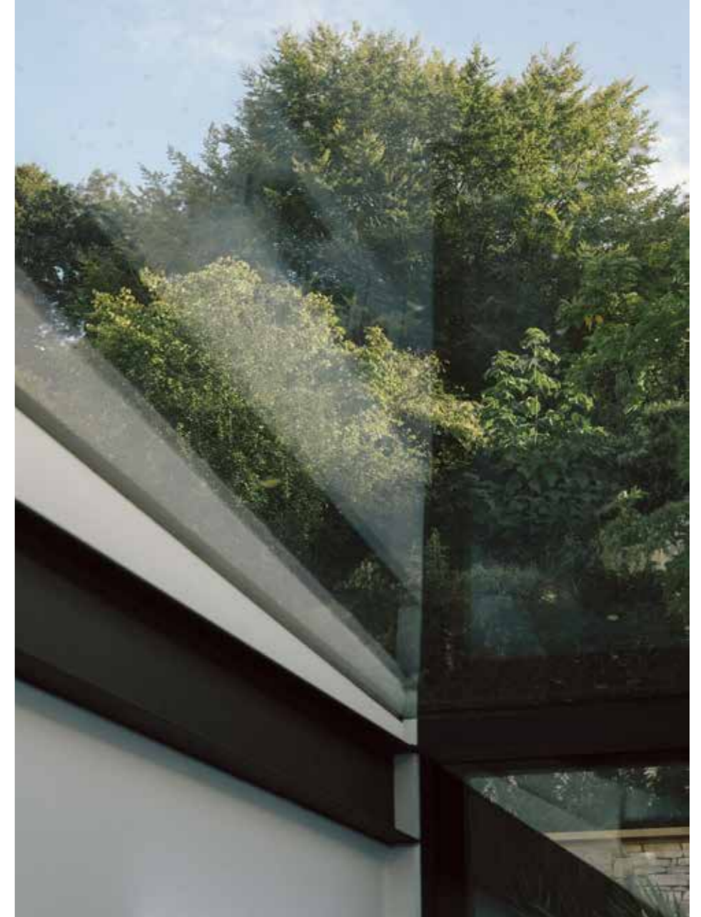
INTERIOR DETAIL : EXPOSED STEEL & STRUCTURAL GLASS
