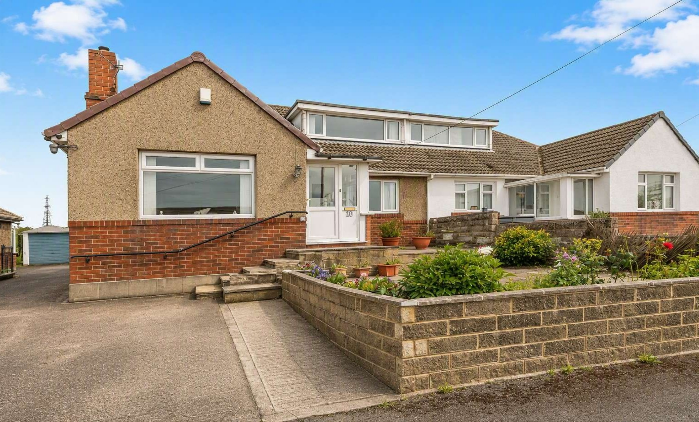
West Lodge Crescent, Ainley Top Huddersfield HD2 2EH
