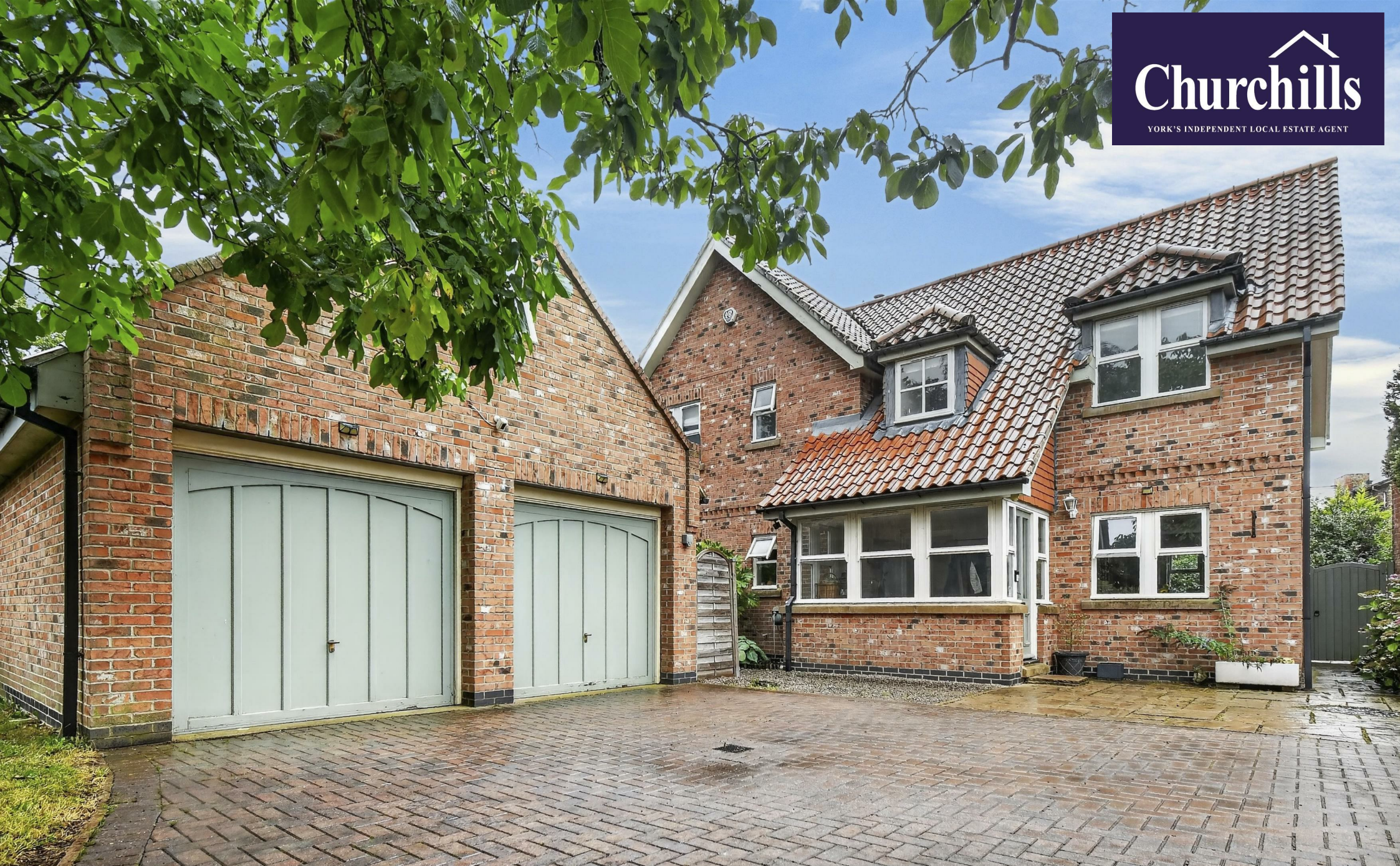
Walnut House Moorlands Lane Tollerton York, YO61 1QR £700,000
