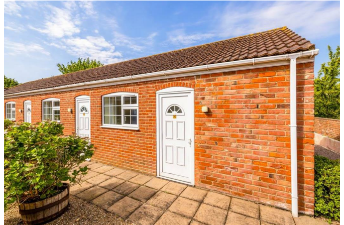
Letting Room 8 11'6" x 12'11" (3.53m x 3.94m)
