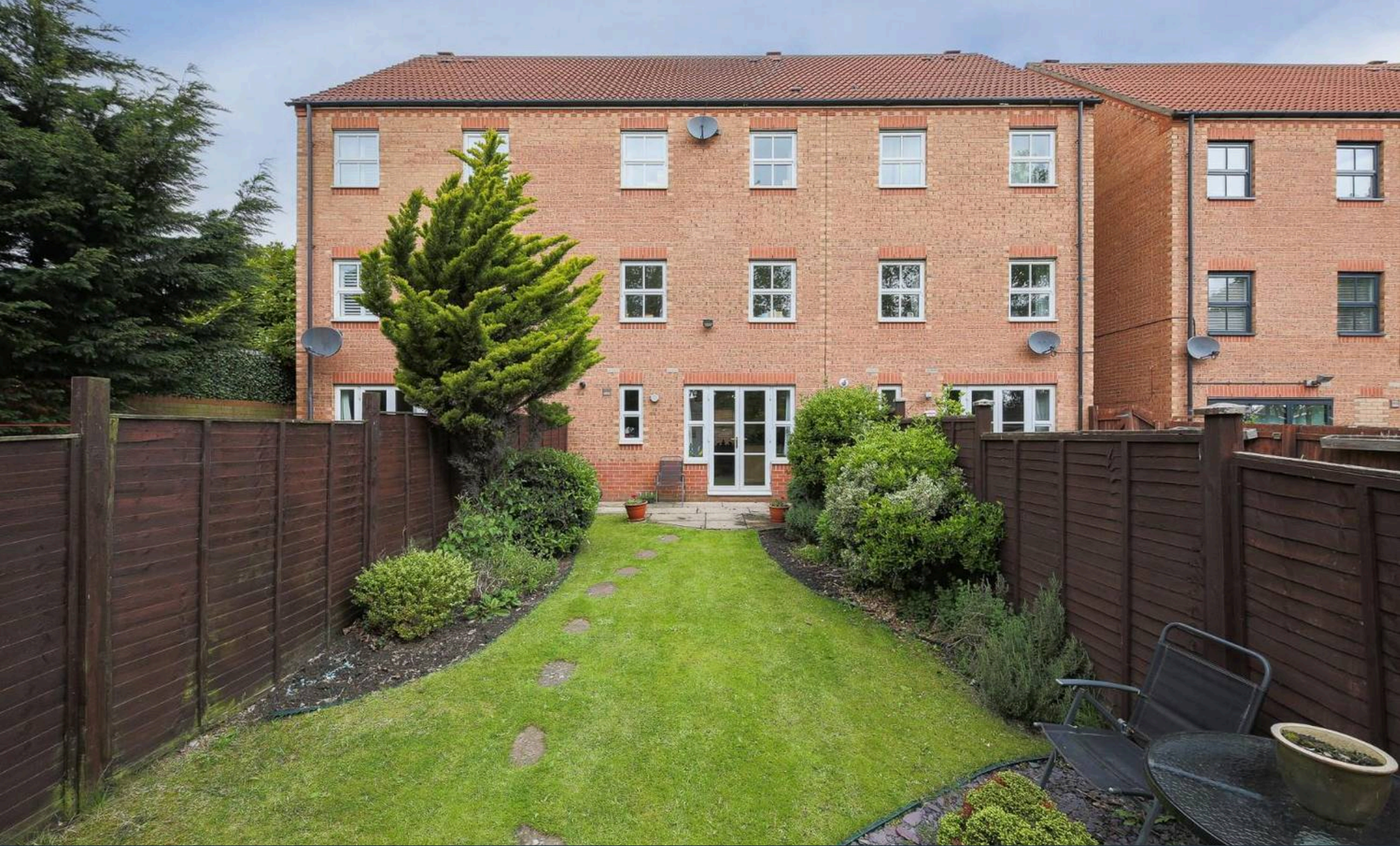
2 Backworth Court, Backworth Newcastle Upon Tyne
