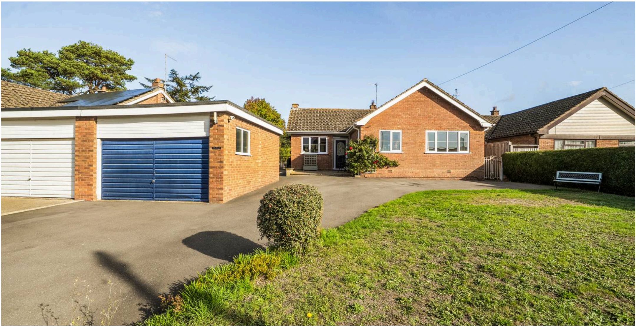
The Croft Crown Lane, Defford Worcester
