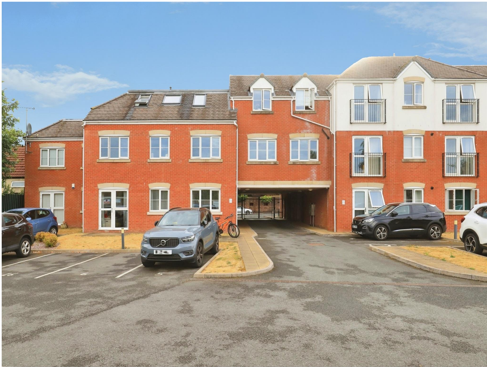
Terreno Court Apartments High Street,Amblecote Stourbridge DY8 4FD
