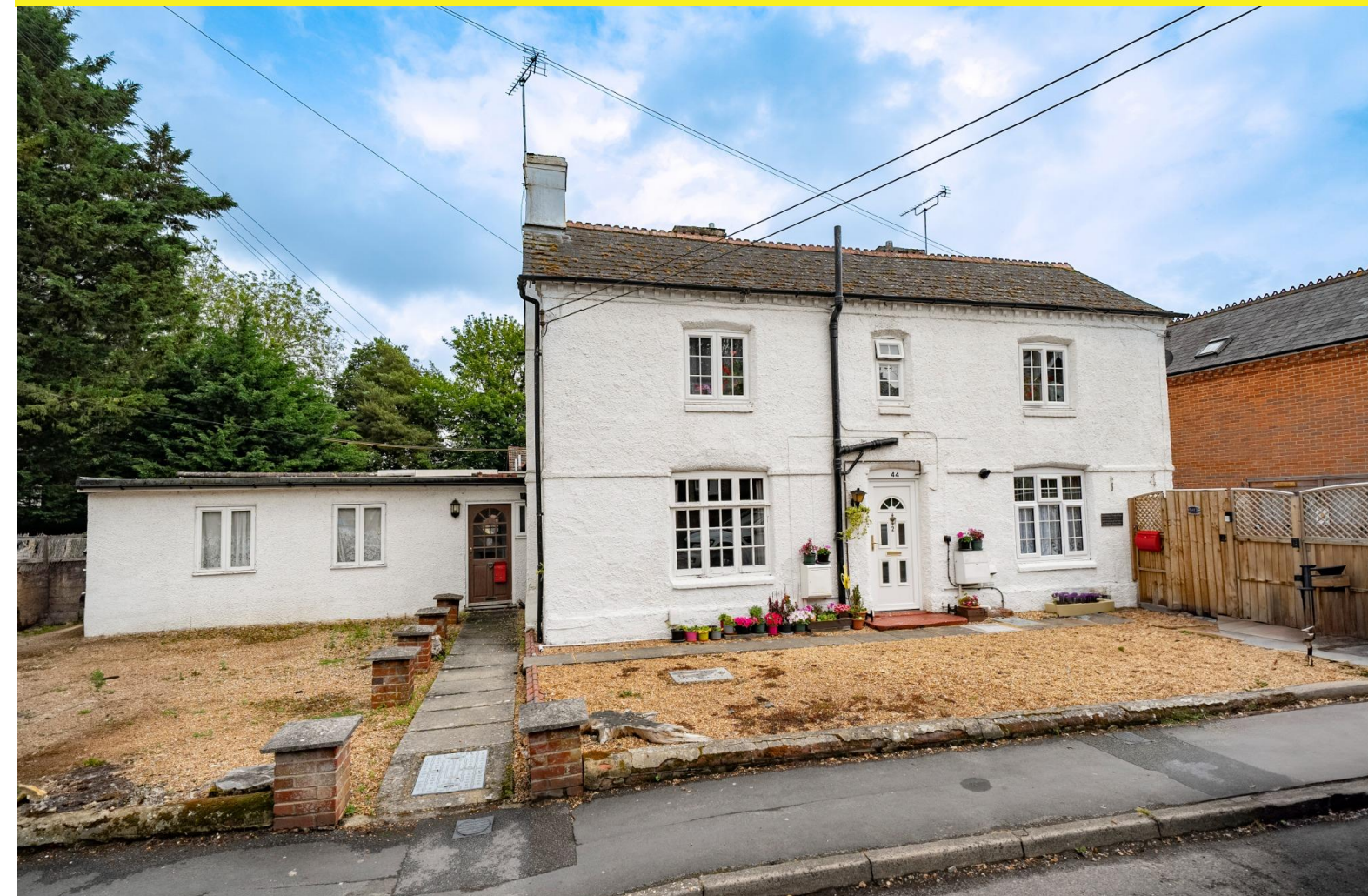
Junction Road, Andover
