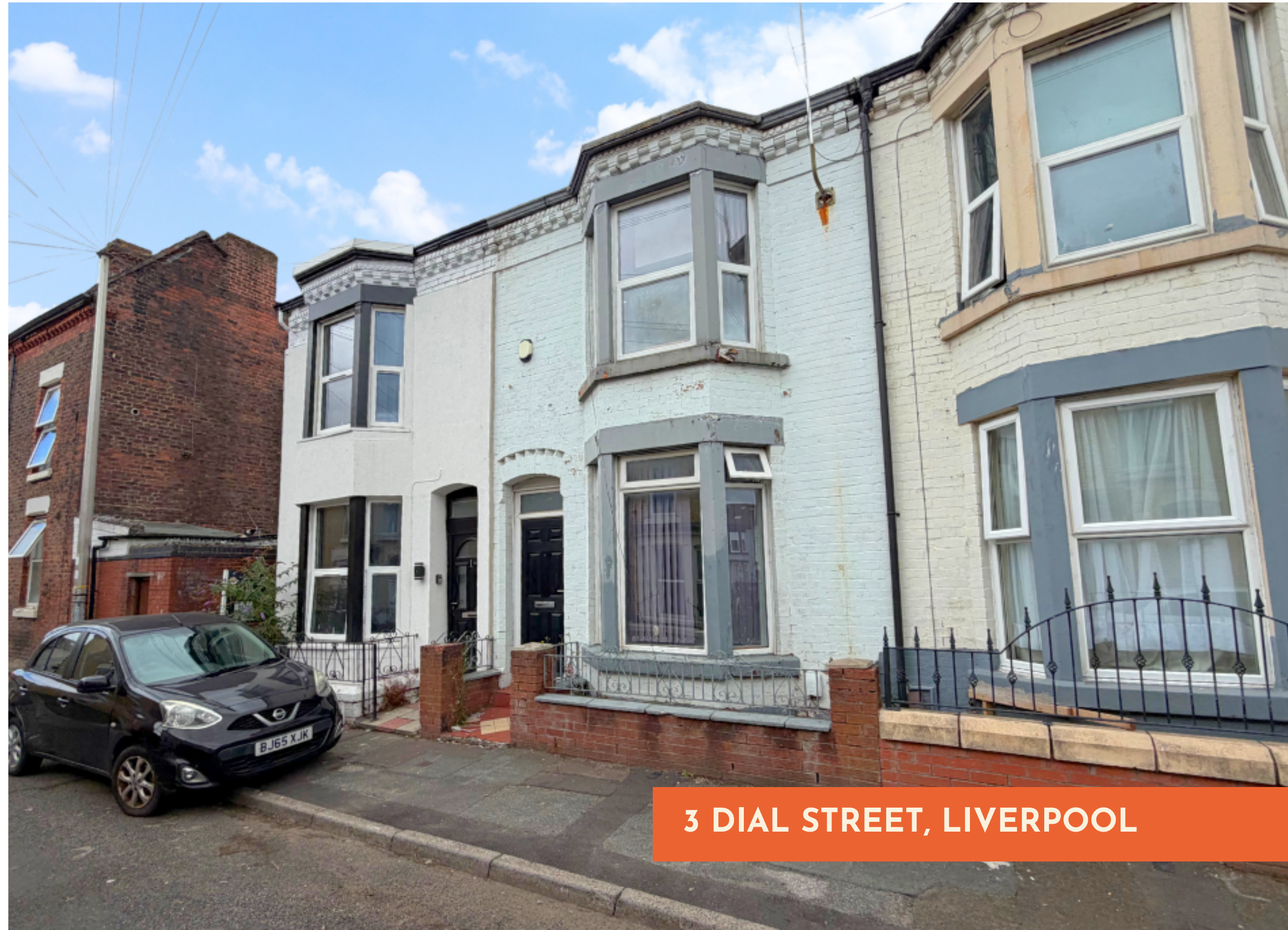
FRONT OF BUILDING
