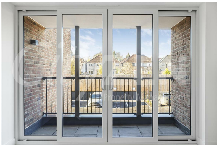
DOORS OUT TO BALCONY
