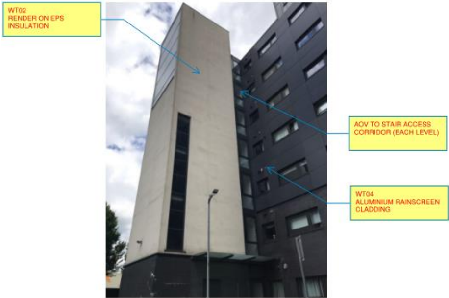
Figure 7—3 Cladding systems adjacent to stair cores
