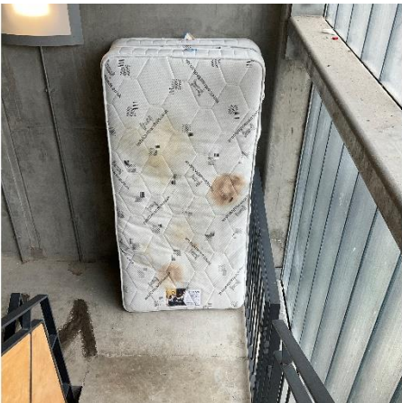
Figure 9—2 Combustibles stored within stairwells
