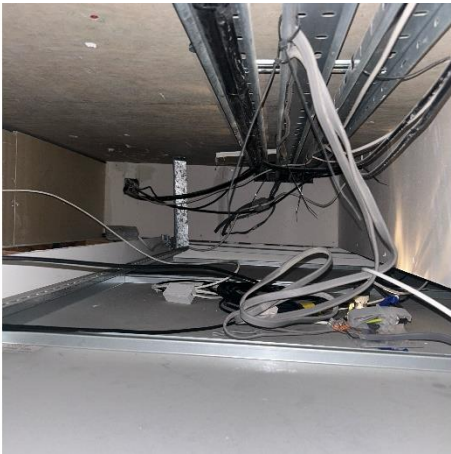
Figure 9—4 Firestopping required
