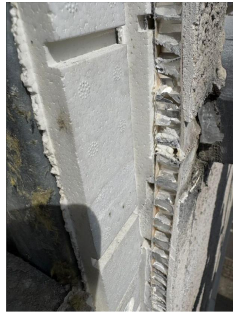
Figure 5—5 Evidence photo 4. Polystyrene packer installed to face of SFS
