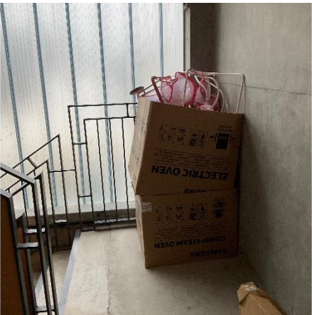
Figure 9—1 Combustibles stored within stairwells
