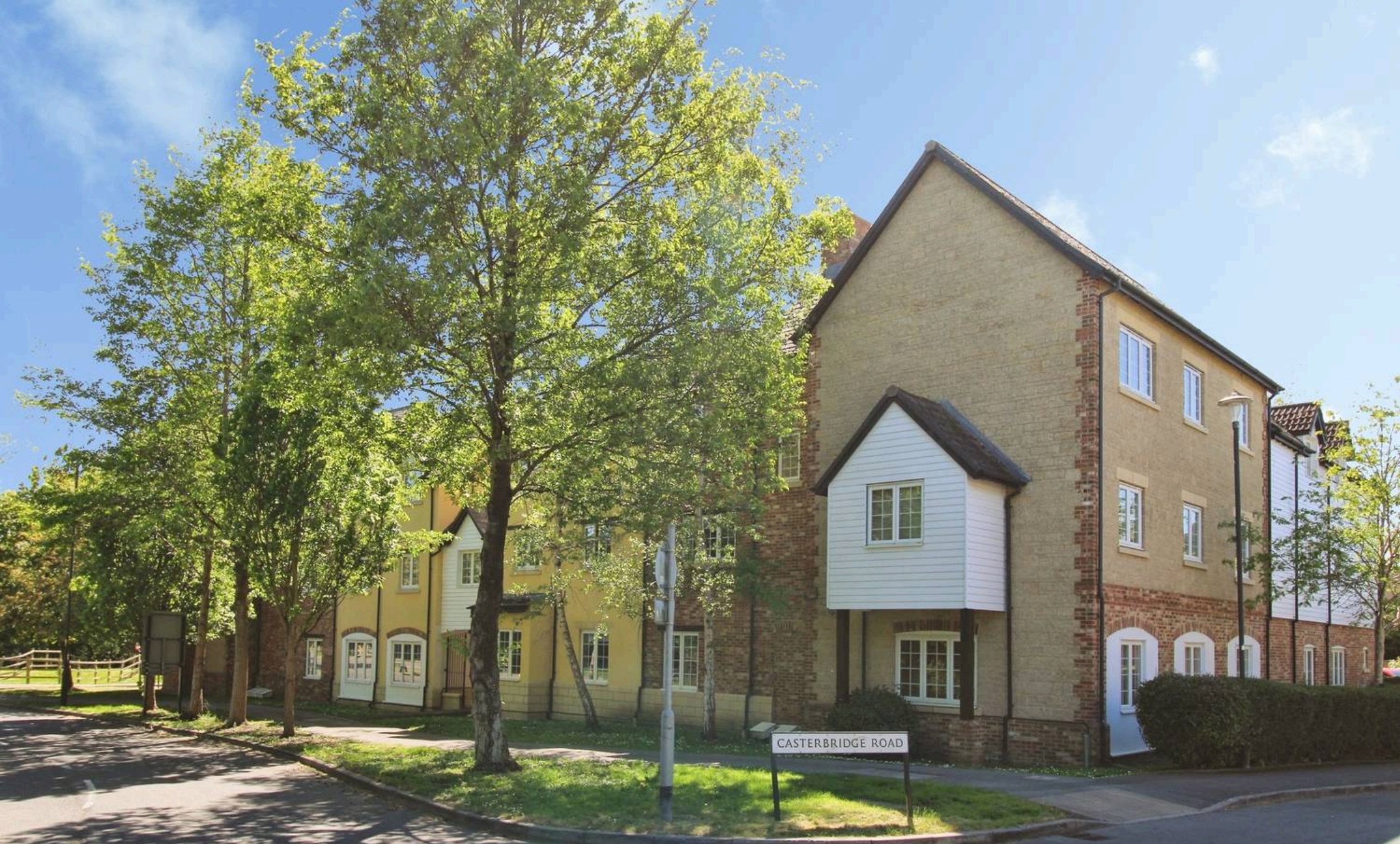
9 Livinia House, 1 Maybold Crescent Swindon
