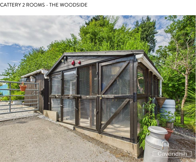
2 cat rooms to the right hand side of the main building.
