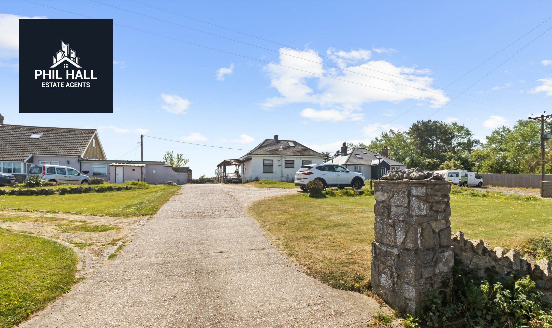
Howard Cottage Eastbourne Road Pevensey, BN24 6DT
