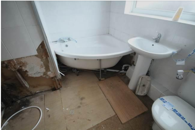
BATHROOM: Radiator, double glazed window, w.c., wash hand basin, corner bath and space for a shower cubicle to be fitted.
