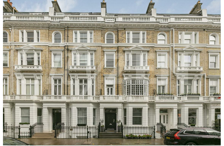
EXTERNAL OF BUILDING
