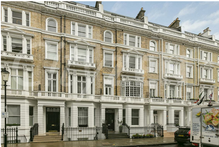
EXTERNAL OF BUILDING
