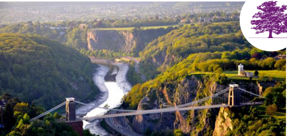
Suspension Bridge 15 Minutes
