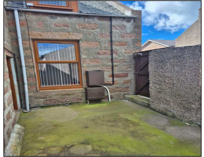
Enclosed Courtyard & Decking Area
