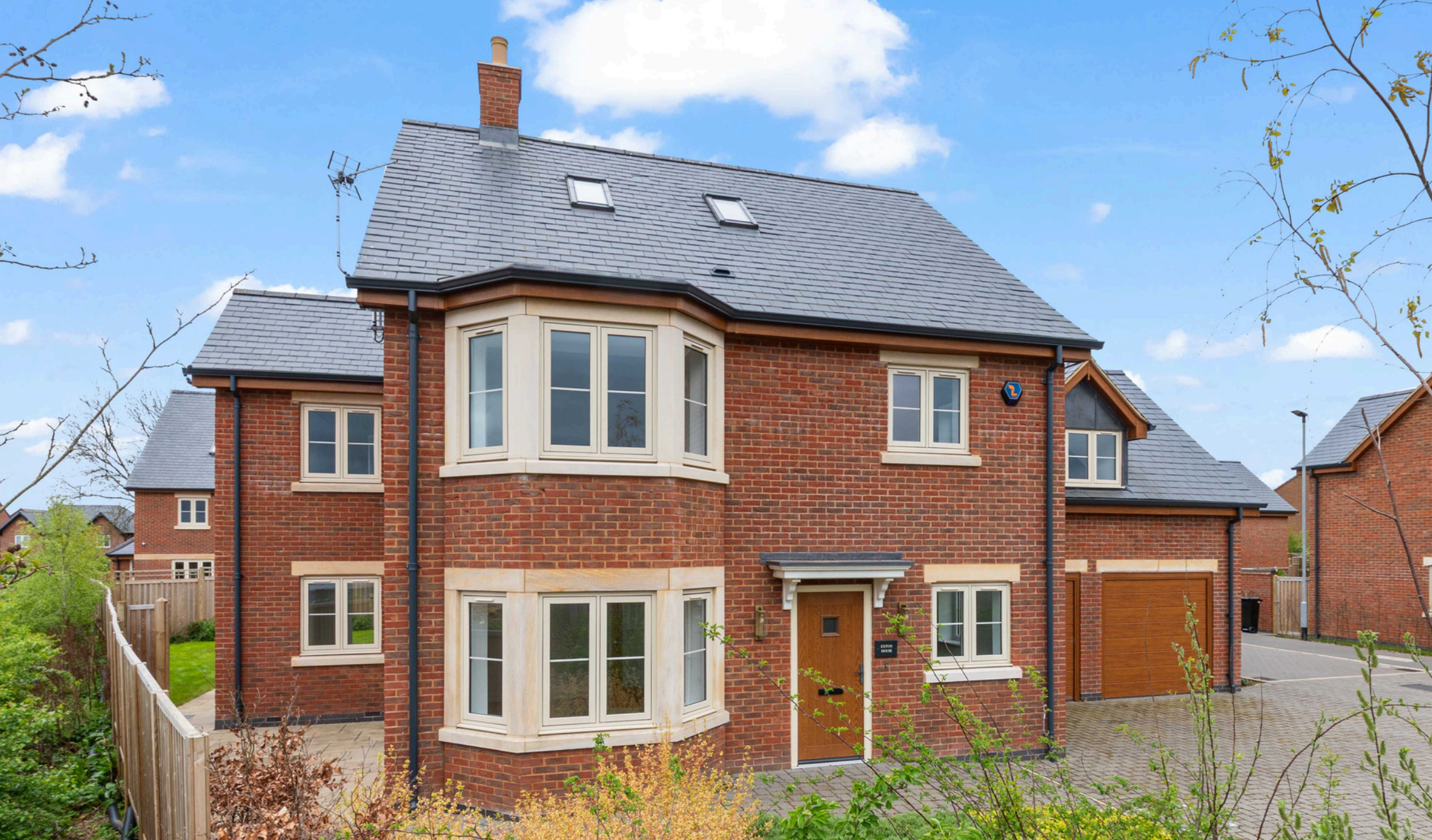
EXTON HOUSE PLOT 7, UPPINGHAM PLACE
