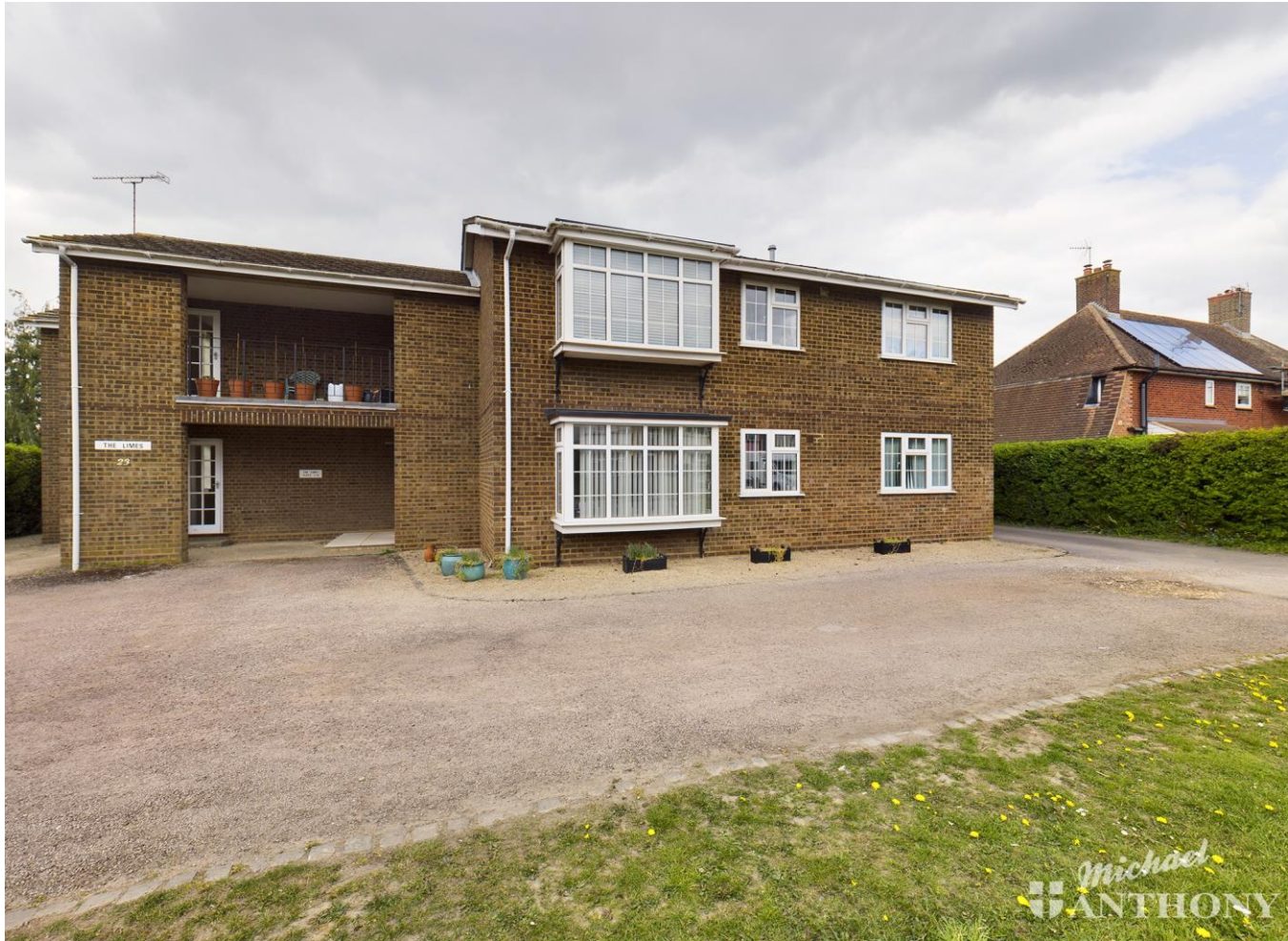
View of block
