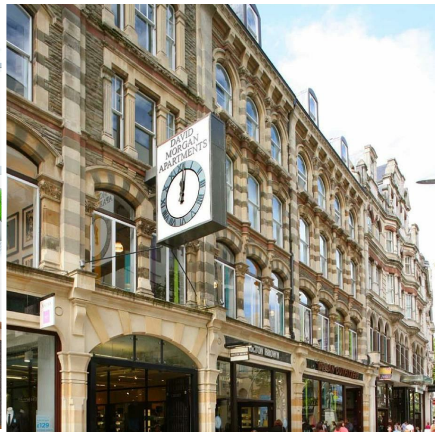
David Morgan Apartments, Barry Lane, Cardiff
