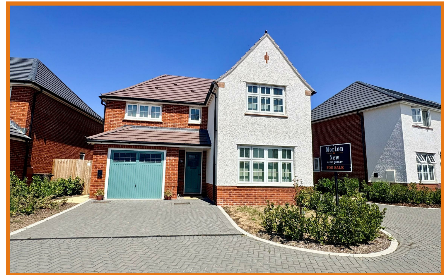
Tile Terrace Gillingham
