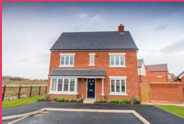
Great Denham, Bedfordshire
