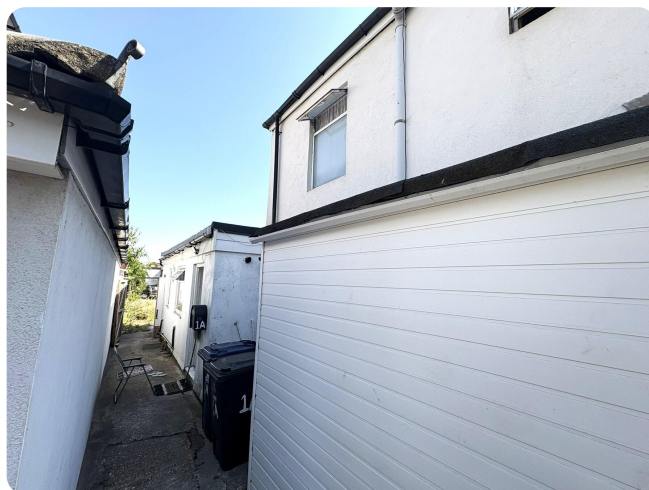
SIDE ACCESS — ENTRANCE TO 1A
