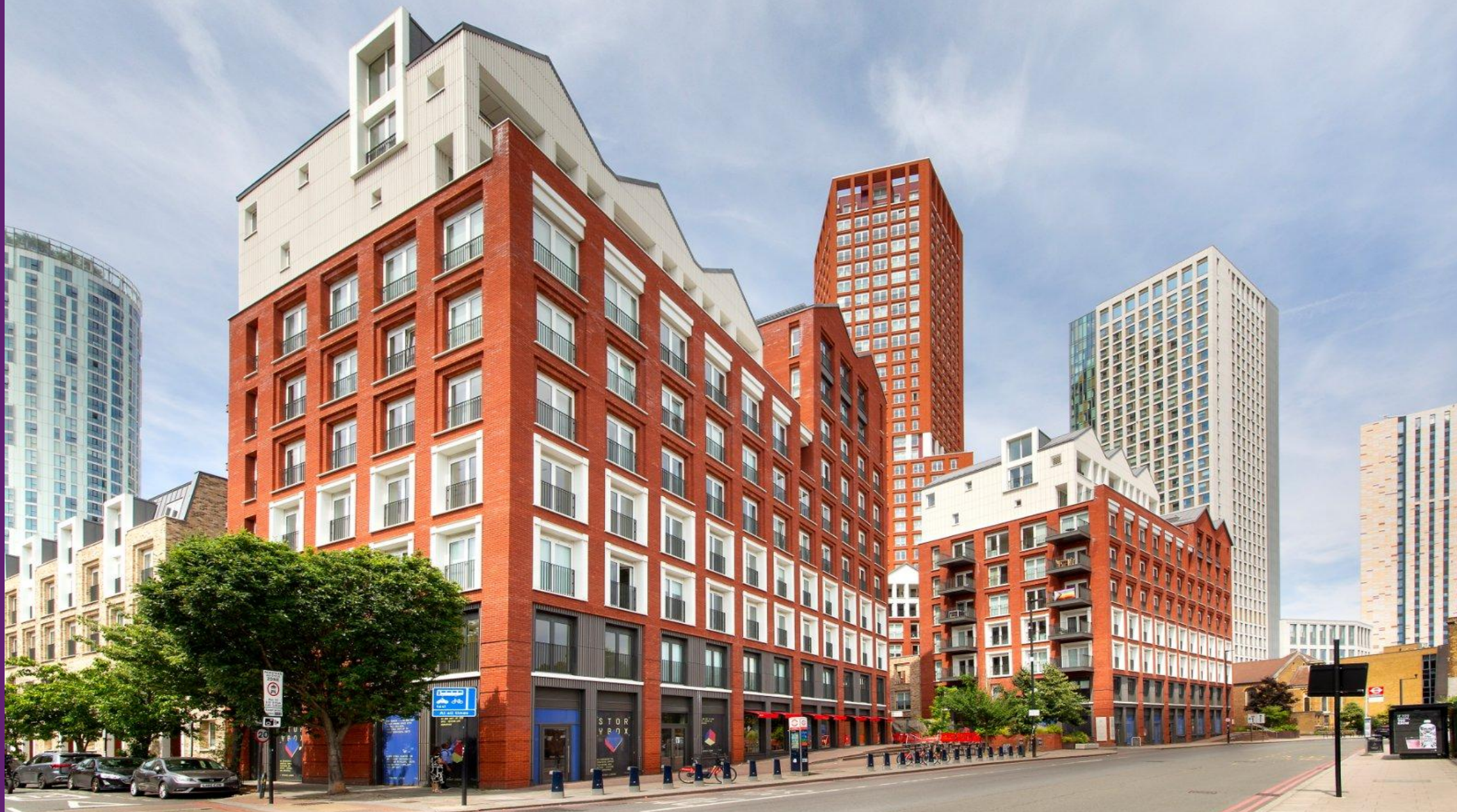
Exchange Gardens London, SW8
