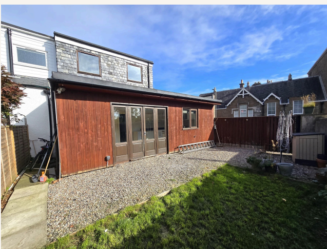
EXTERNAL REAR 4 EAST SCHOOL ROAD (1)
