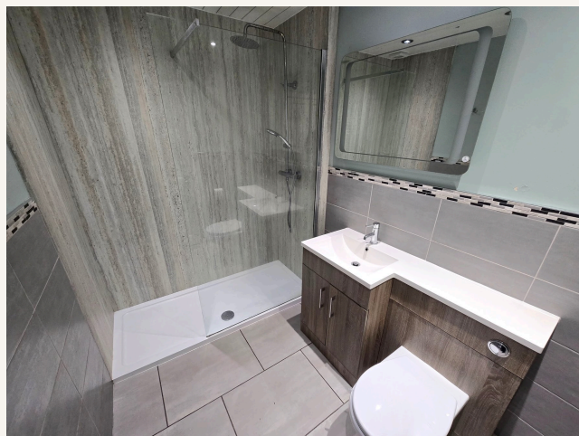
BATHROOM 4 EAST SCHOOL ROAD (1)
