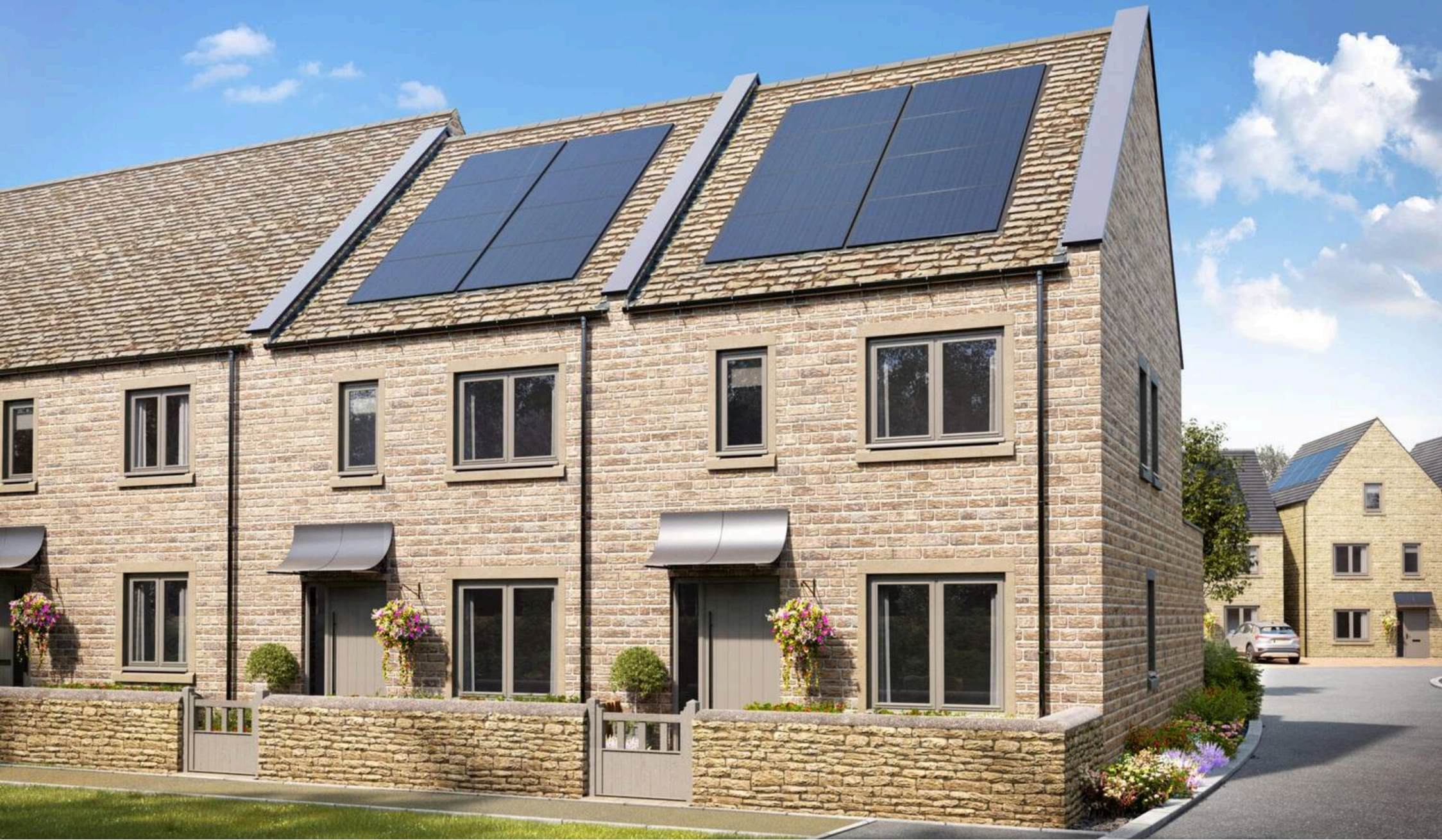
The Bourton, London Road Tetbury
