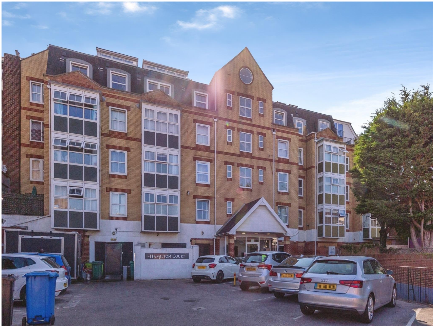
Hamilton Court, Ashby Place, Southsea PO5 3NP
