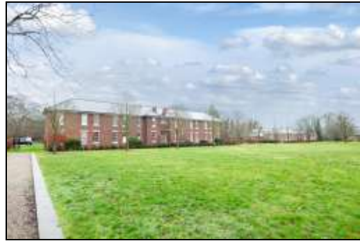
View to Rear of Block
