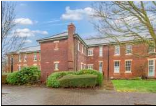
Side View of Building
