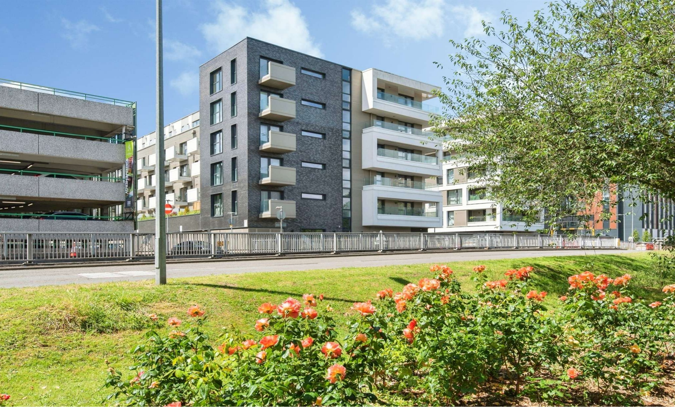
Mulberry House Park Place, Stevenage SG1 1BH
