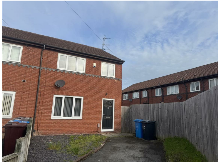
With off road parking for several cars.
