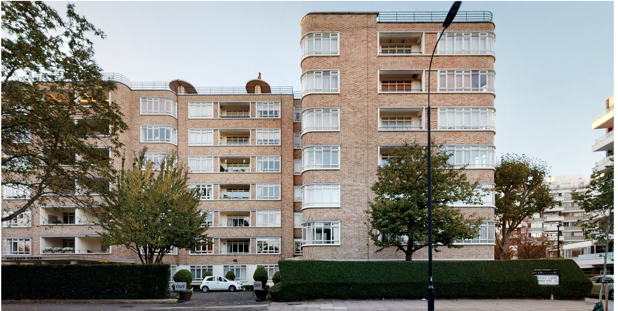
VICEROY COURT, PRINCE ALBERT ROAD, St John's Wood NW8
