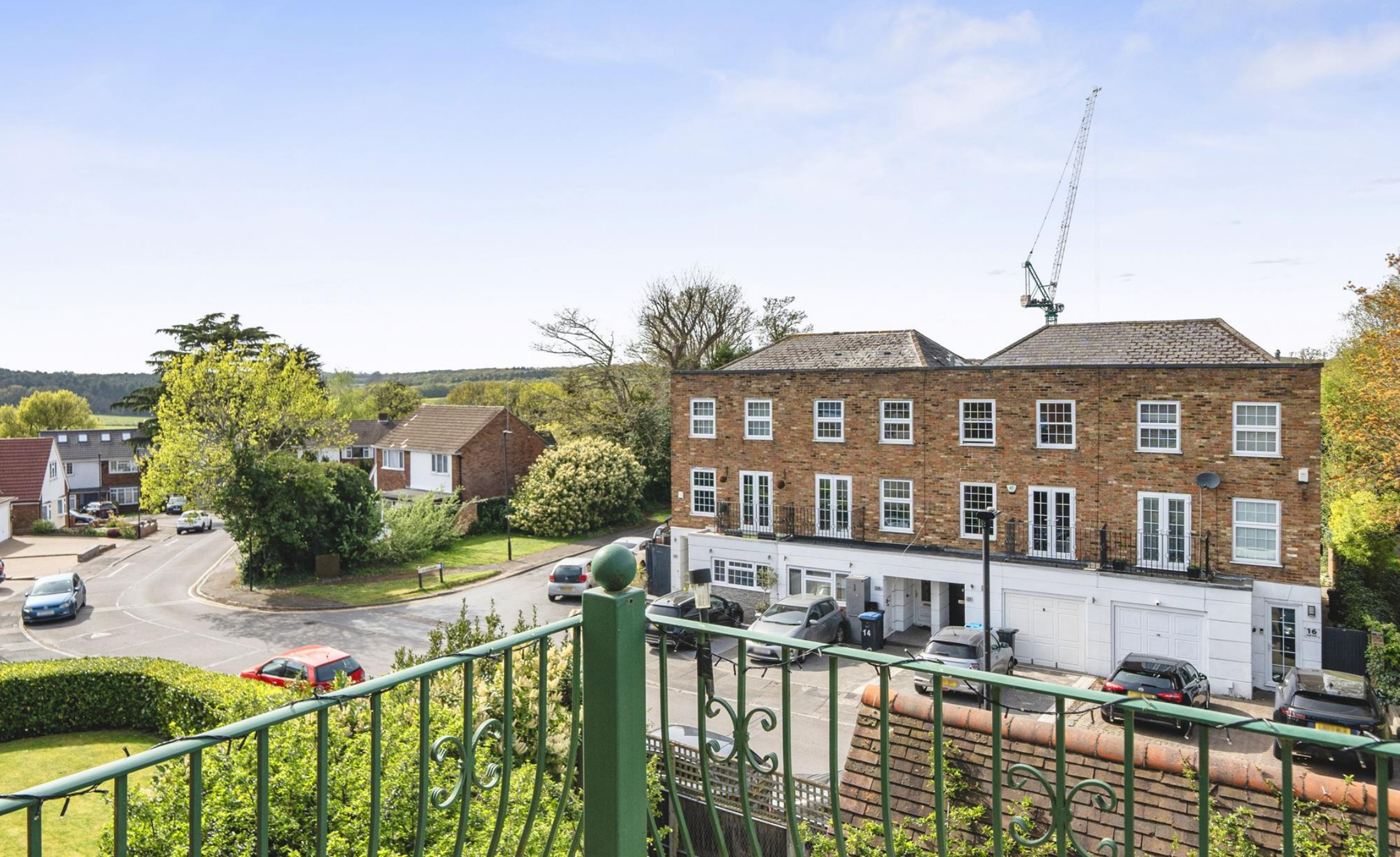
Holywell Lodge, The Ridgeway, Enfield, EN2 8JN
