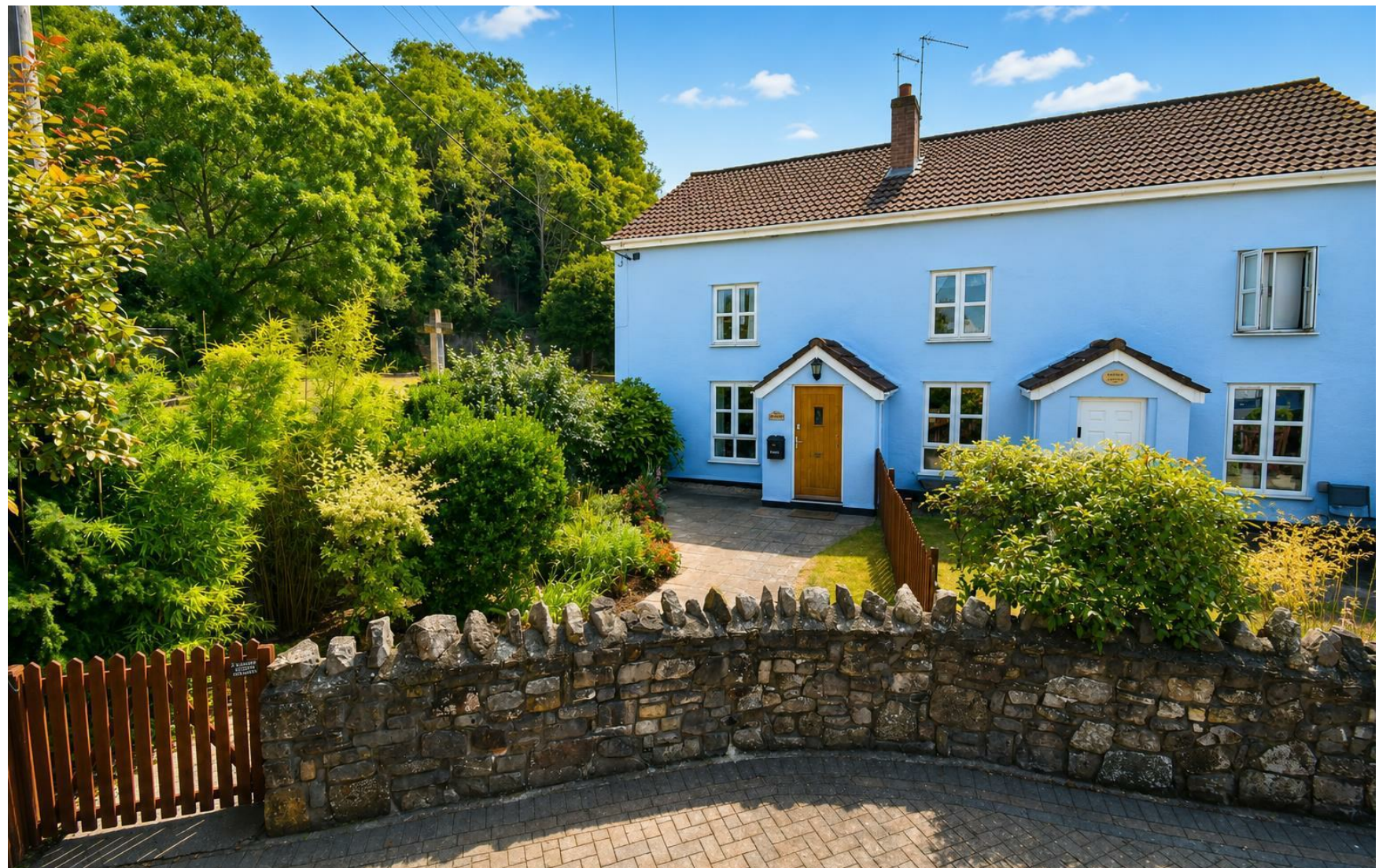
MARSH COTTAGE MOORHOUSE LANE
