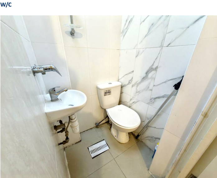
sky light window - wall mounted wash basin - low flush w/c - tiled walls - tiled floor covering.
