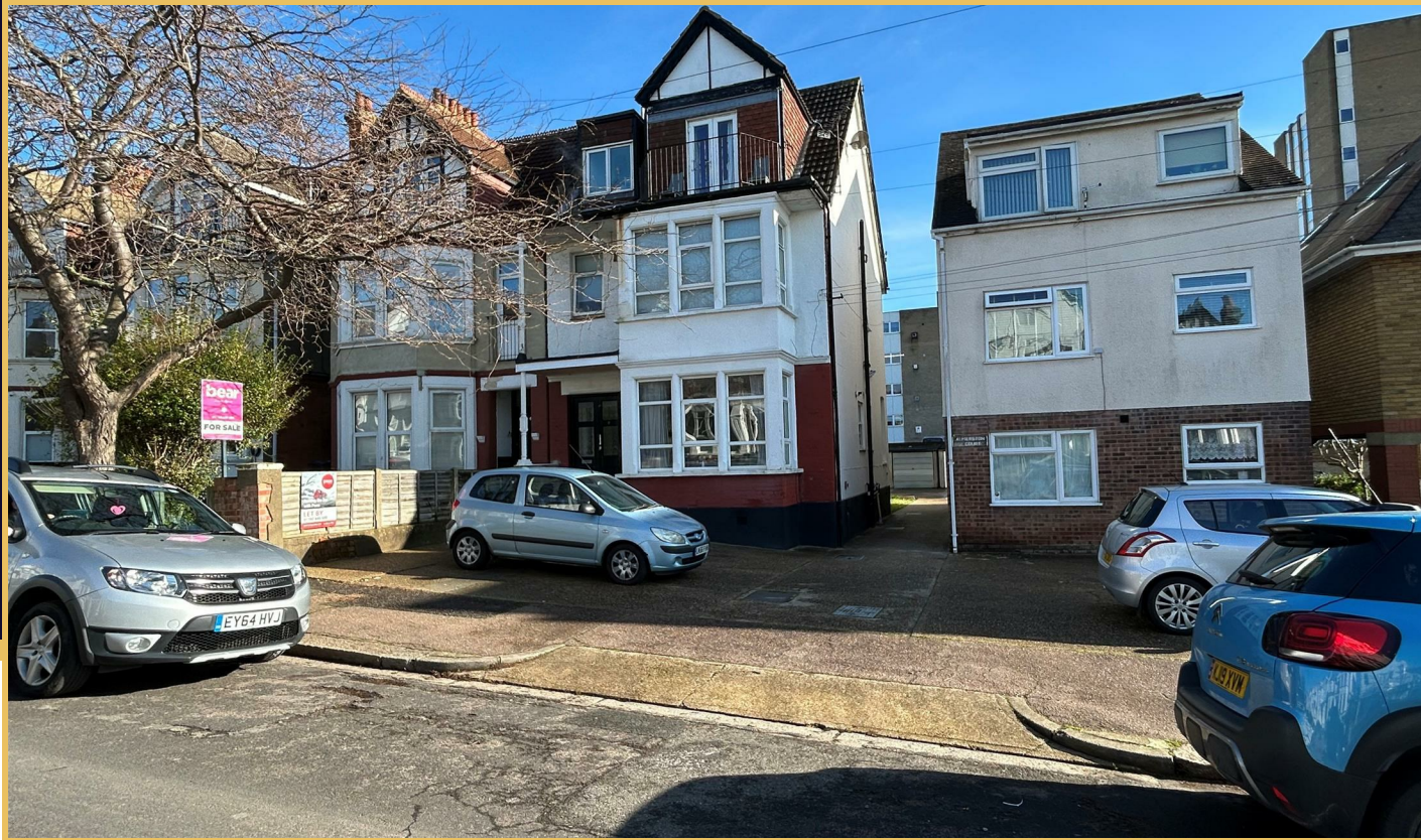
Palmerston Road , Westcliff-On-Sea SS0 7TB
