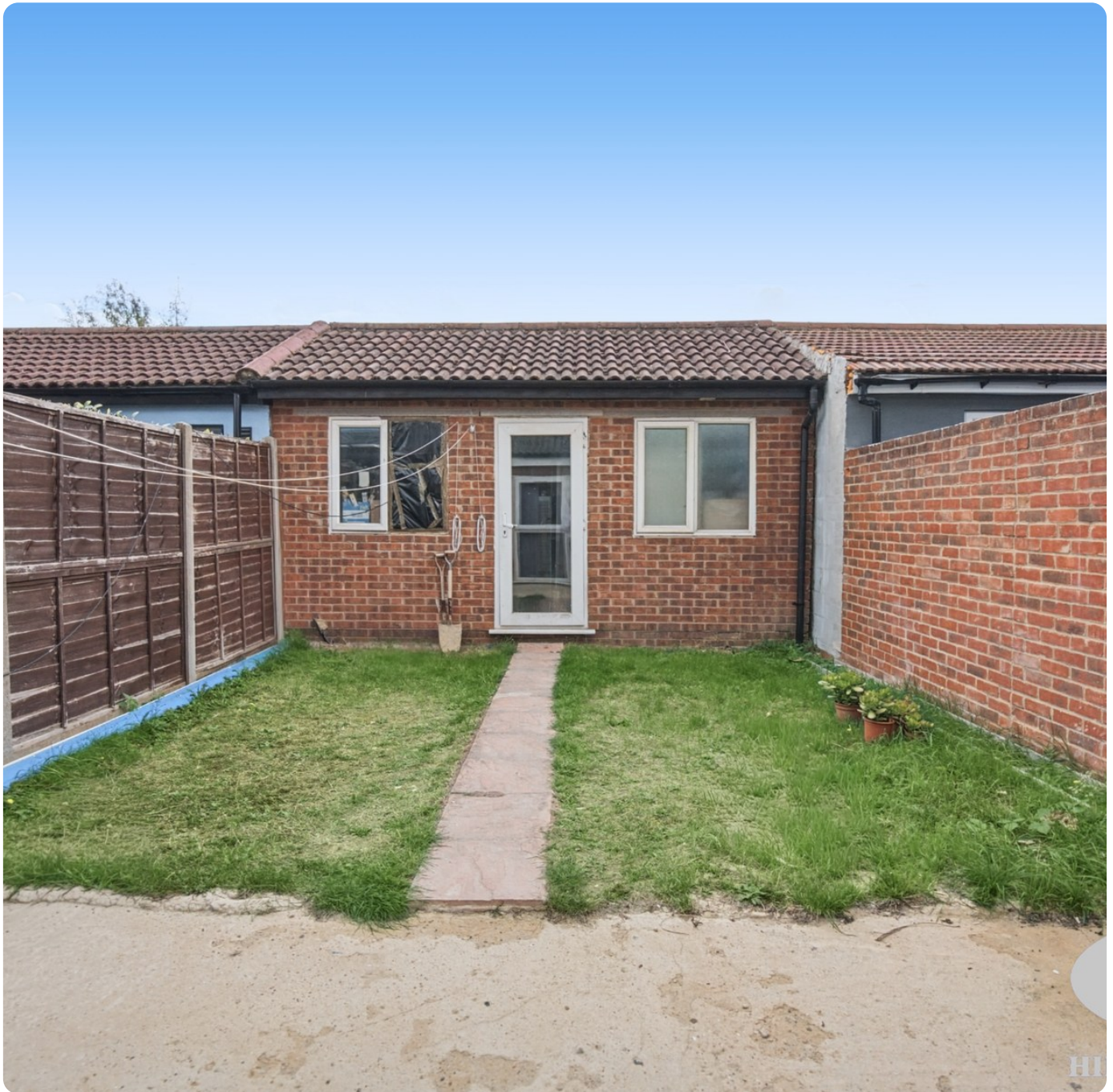
ANNEX & SHOWER ROOM
