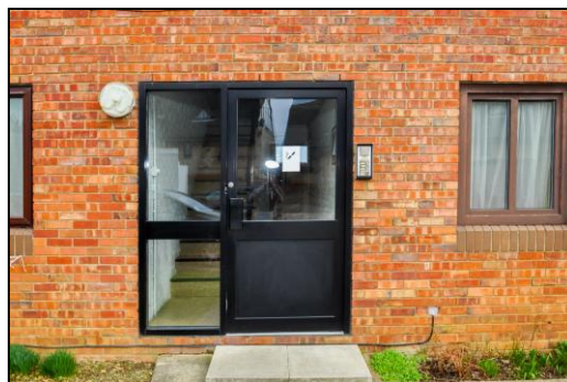
Communal front Door with Intercom
